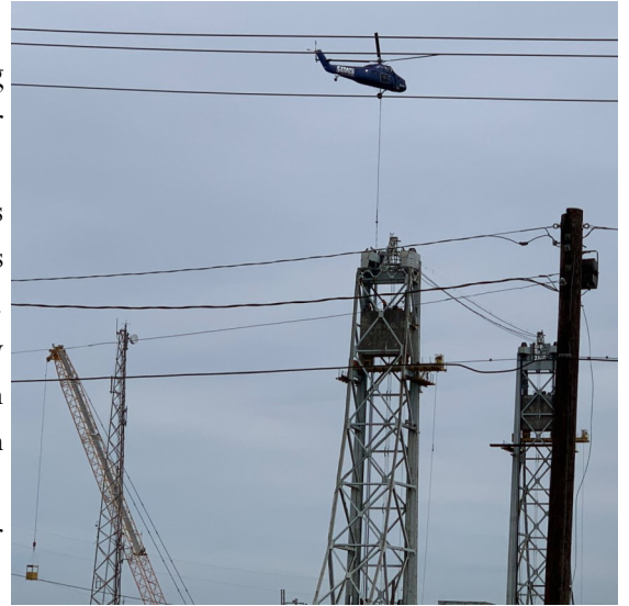
KCS vertical lift bridge repairs being made in October, 2019.
