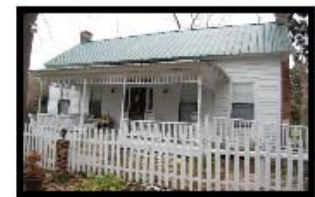
W.T. Colmesneil House
